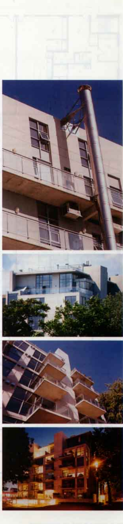
Top right: the frankly exposed services on the west side. Above right: a view of the penthouse, overlooking the park. Above right: balconies flanking an elevator tower on the park side. Right: an evening view from the park.
