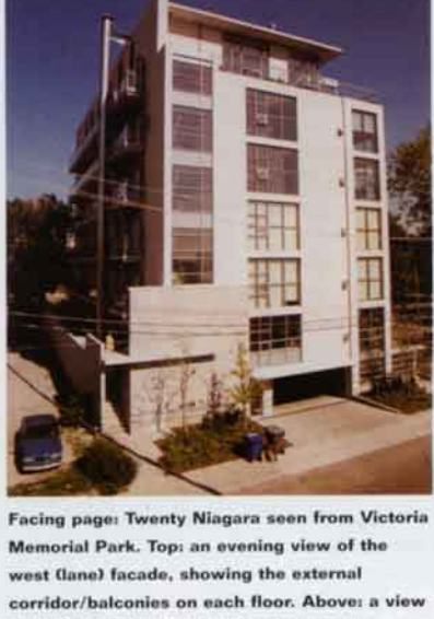
Facing page: Twenty Niagara seen from Victoria Memorial Park. Top: an evening view of the west (lane) facade, showing the external corridor/balconies on each floor. Above: a view from Niagara Street, showing the parking access and stairs from the first floor apartment deck. Above right: the tower form at the building's north end.
