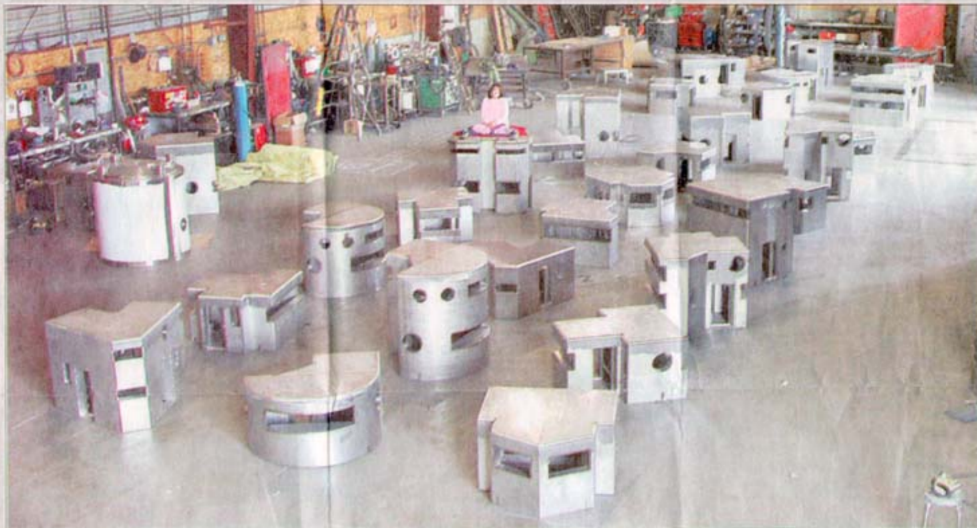
Radioville, a miniature city under construction at Keating Industrial Park, is destined to grace a Toronto plaza development. Roland Brener photo
